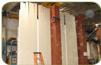
Octaform Finished Panels were slid into the 2" connectors.
