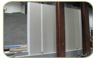
The wall was left to cure for a week prior to testing.
