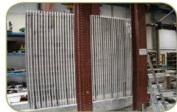
2" connectors slid into H-connectors. Dowels were drilled into the concrete footing as anchors. Rebar was added.
