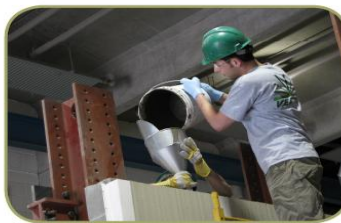
Custom grouting mixture supplied by Vector was placed into the form.
