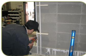
H-connectors were drilled into the wall with a 6" spacing between connectors.
