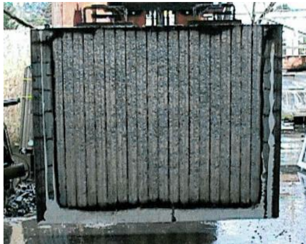
Exposed Octaform Wall After Fire and Hose Stream Tests
