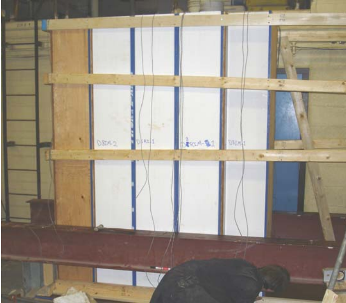
Figure 2.5 Bracing system for the specimens
