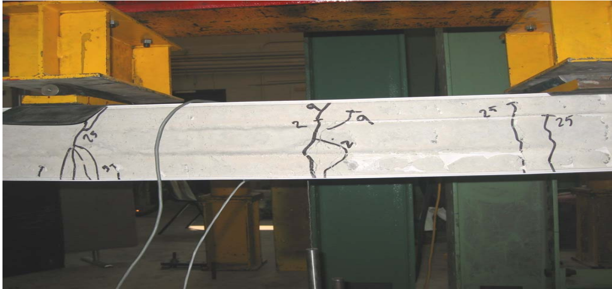
Figure 3.4 Typical crack distribution for encased un-reinforced specimens
