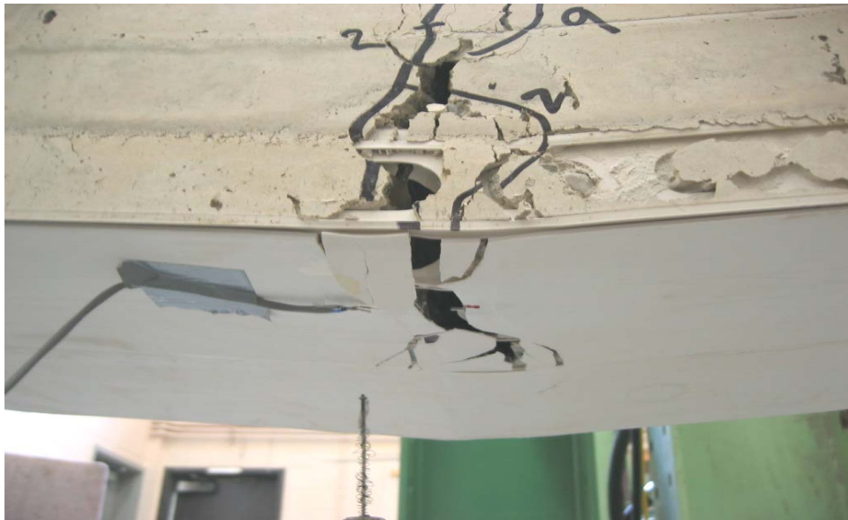
Figure 3.5 Typical rupture of the Octaform panels
