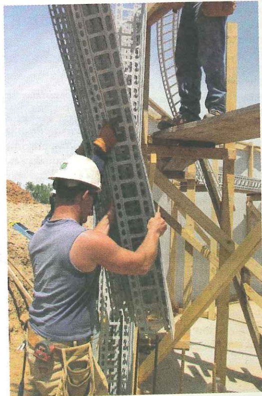
The tanks, which are part of the second stage of the 50-year-old hatchery's expansion program, measure 10 feet high and 36 feet across. They have walls eight inches thick, and were built to help boost the hatchery's trout production.
