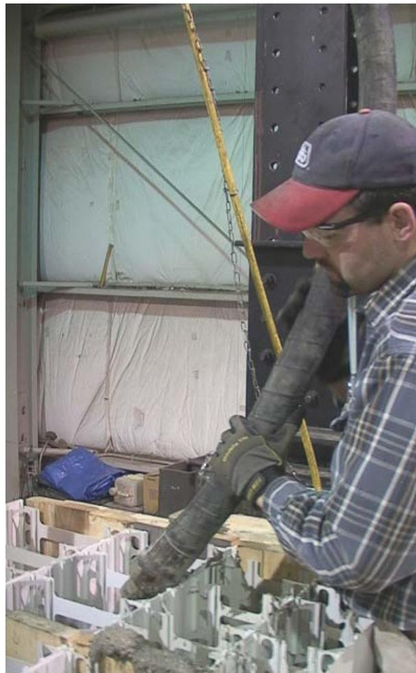
**Figure 6 – Crane and 3" hose from grout pump to place concrete**
