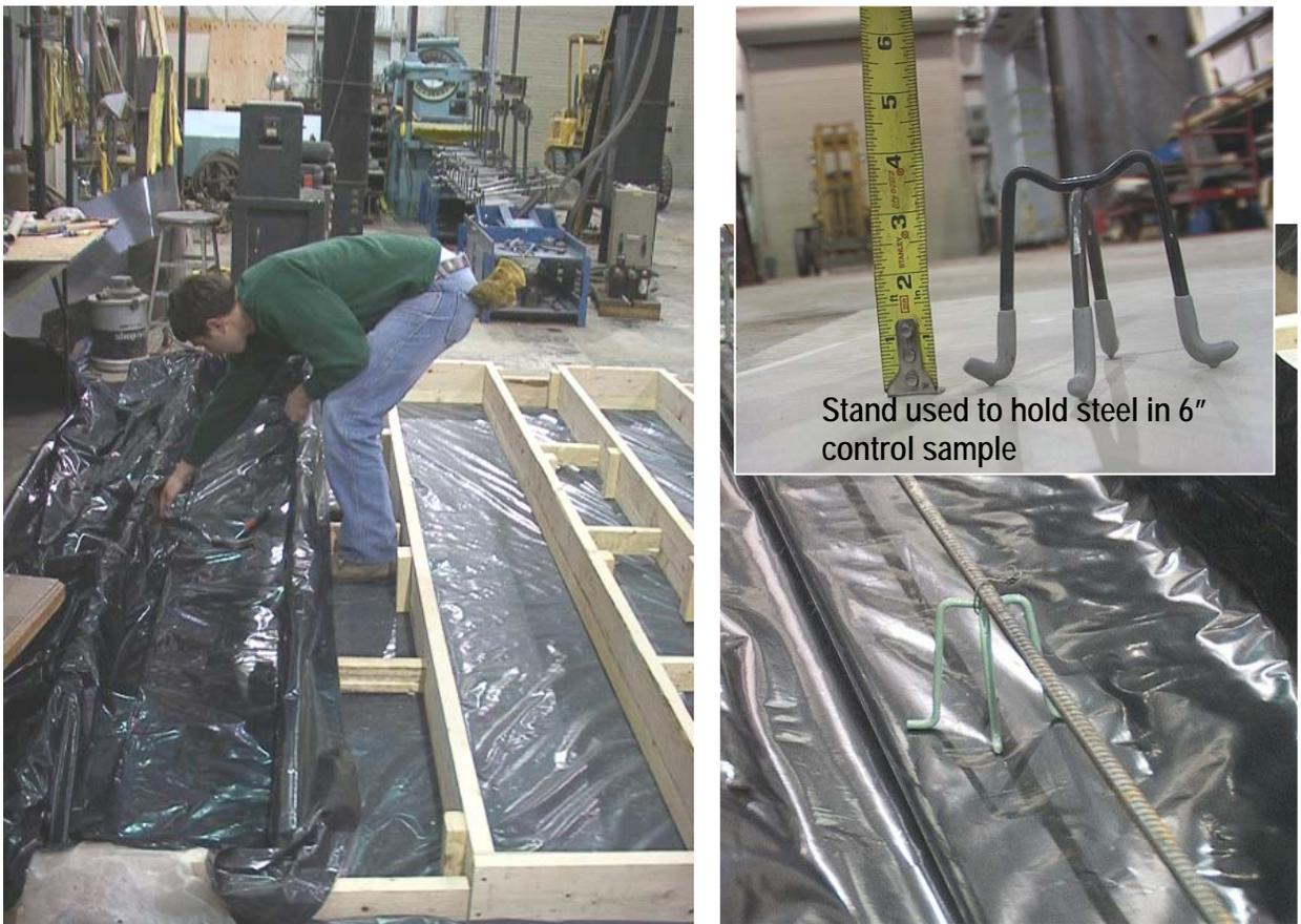
**Figure 5 – Control with plastic and reinforcement in place**
