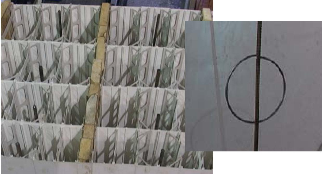
**Figure 4 – Placement of rebar in center of cell using welded rings**
