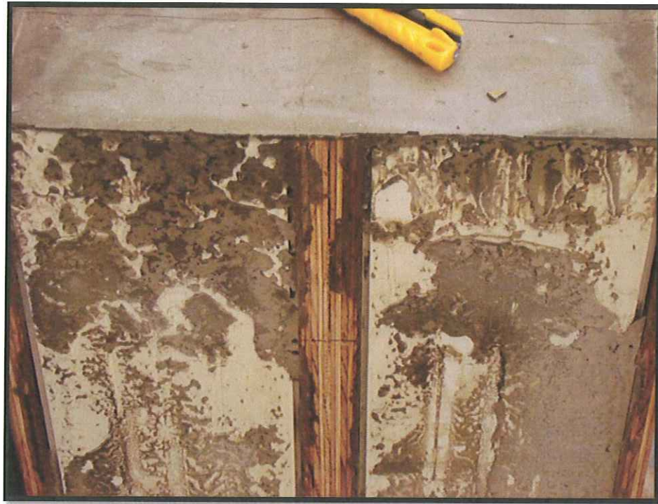
Side view of columns during stripping
